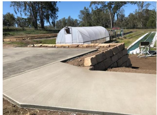
installed, between the tear-drop and the block wall in the image at left. The geotextile underlay and the new pond line designed to Qponics specifications will be installed in early February.
